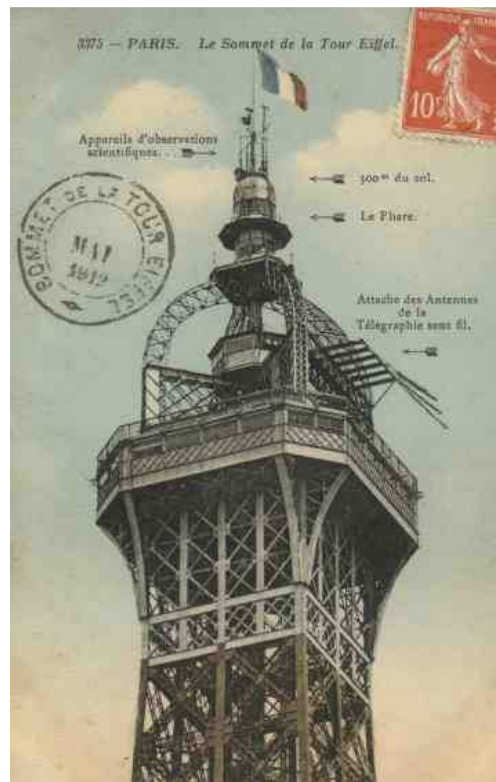
The summit of the Eiffel Tower in 1912 showing the attached antennas (postcard).
